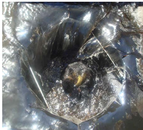
OIL LADEN RUNOFF ENTERING PC+ SEDIMENT BAG THROUGH 24" DIAMETER OPENING
