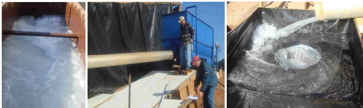
Inside View of Hopper Agitator
