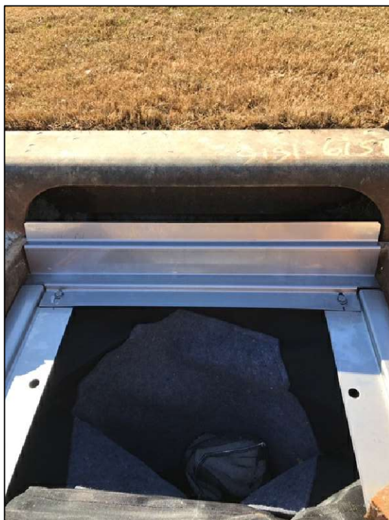
Flexstorm Installed in 2'x3' Curb Box
